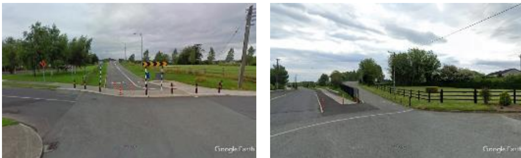
Figure 24. Ploopluck Bridge south (l) and north (r) access points
