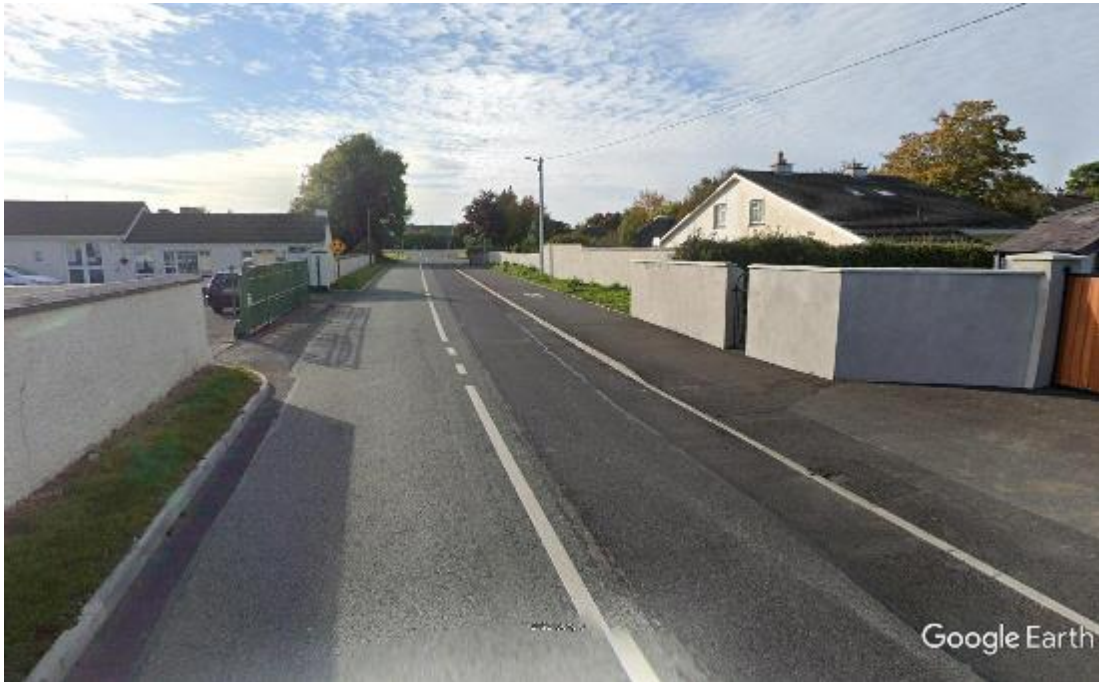
Figure 13. Old Caragh Road looking west to Cois ne Feadain
