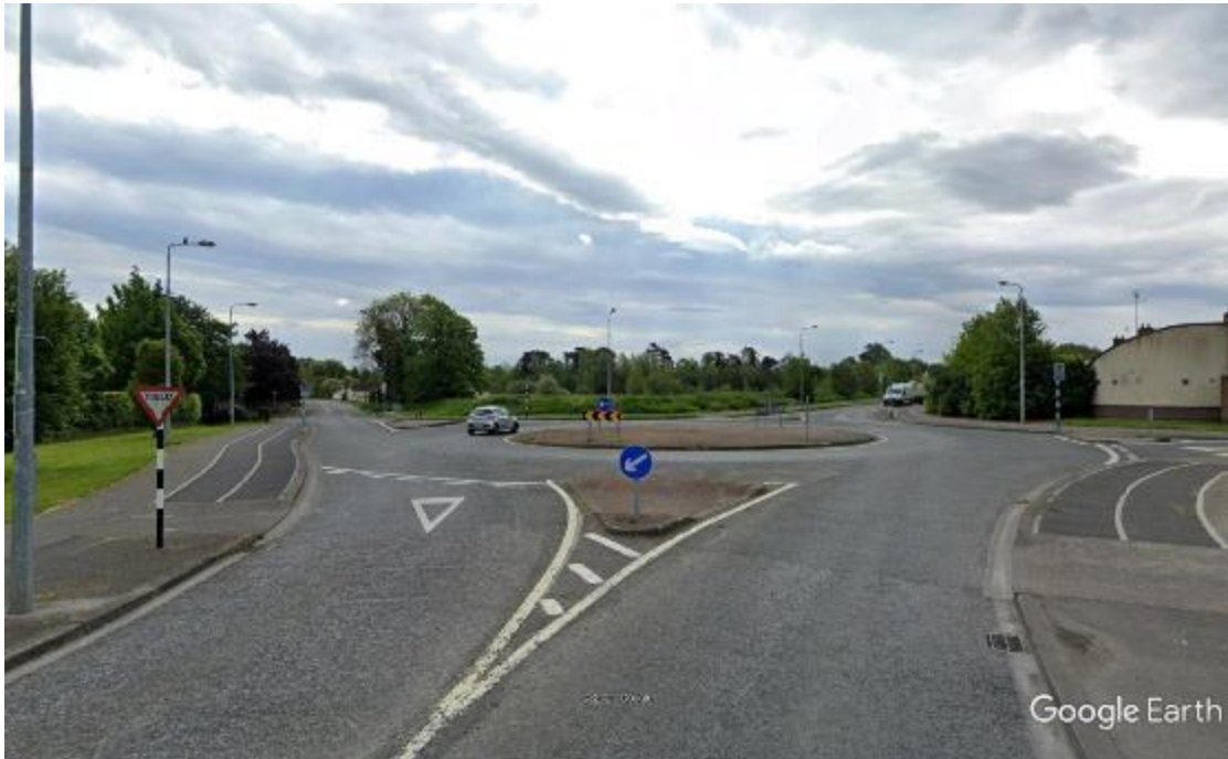
Figure 15. R409 Cois ne Feadain / Old Caragh Road priority roundabout
