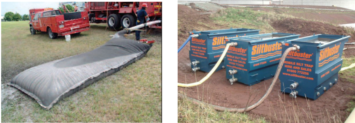
Figure 8 – Typical example of silt bag and temporary settlement ponds
