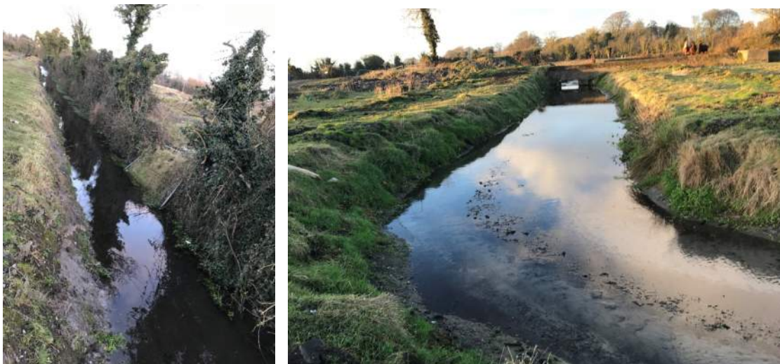
Figure 4 Typical view of existing open watercourse
